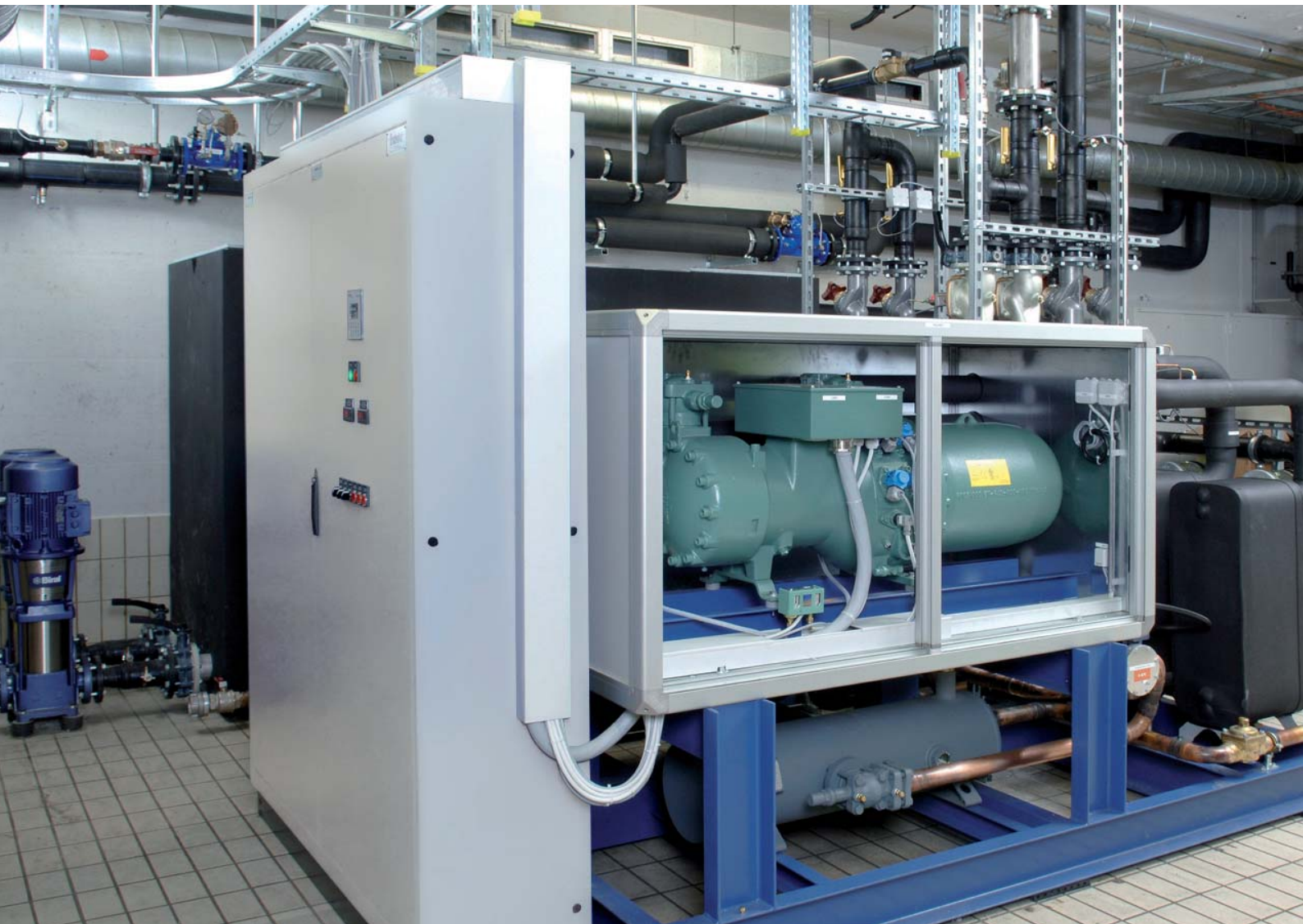
Utilising waste heat from a production process with two KWT heat pumps, each with 400 kW.
