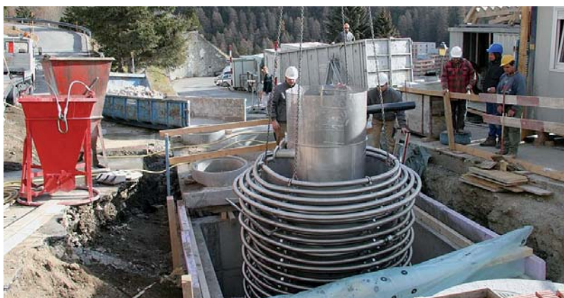
This FEKA waste water pipe is used as a primary source for DHW heating.
