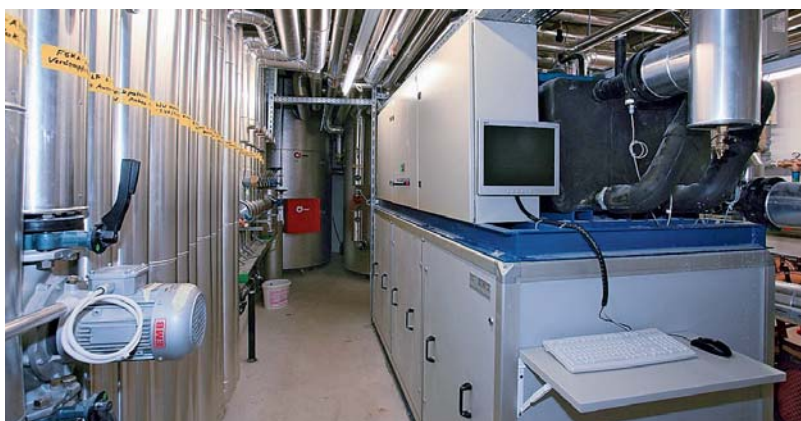
A KWT waste water heat pump with 150 kW output for DHW heating.
